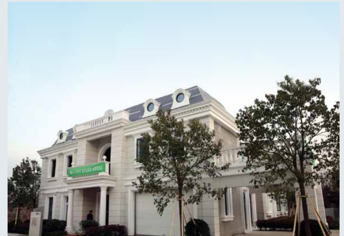
A stand-alone villa, which has been 3D printed by WinSun Decoration Design Engineering Company
